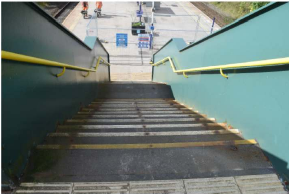
Photograph 6 – View from footbridge onto island platform
