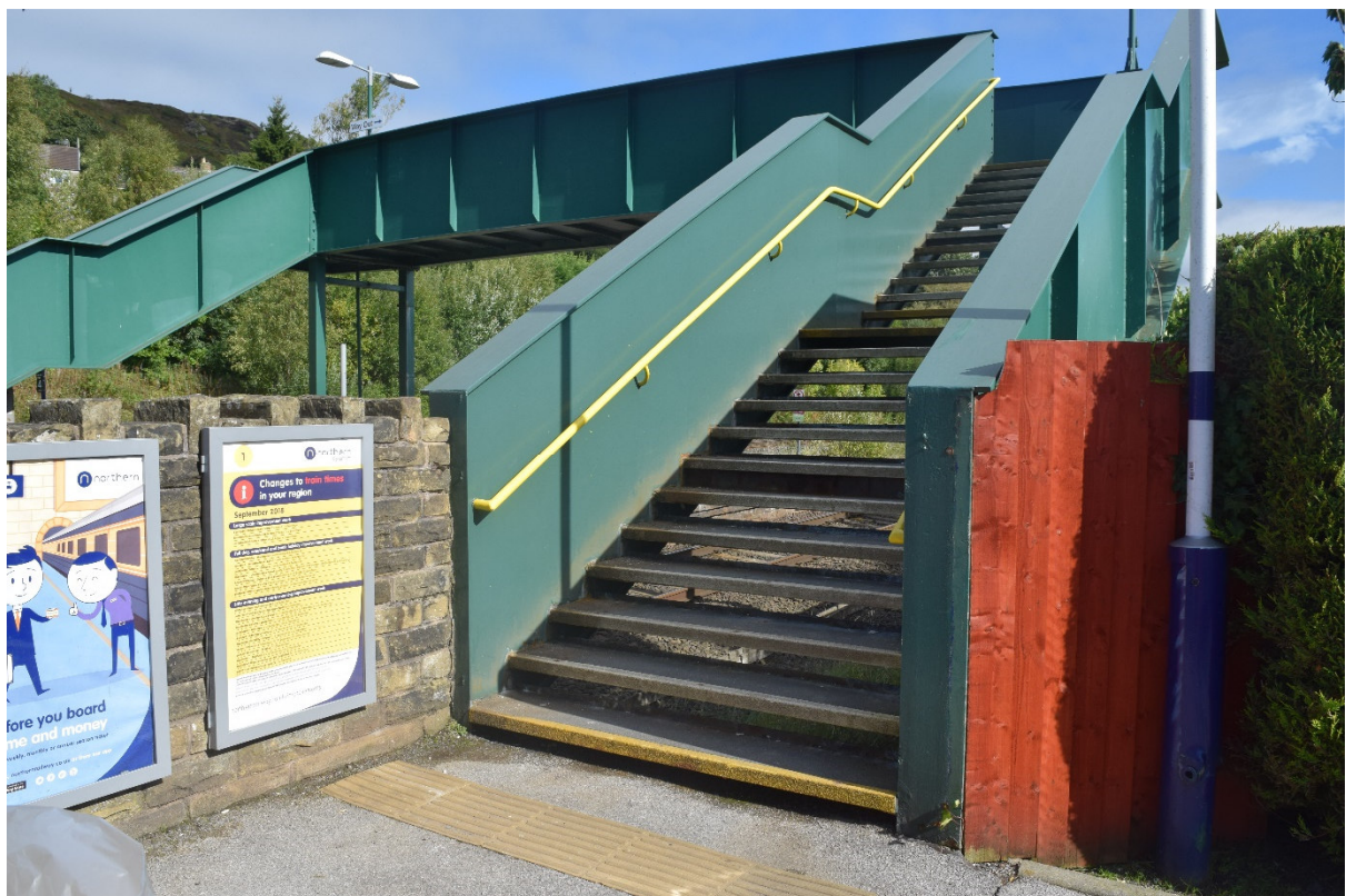
Photograph 4 – Existing Footbridge at Chinley Station
