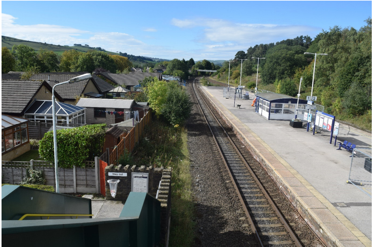
Photograph 5 – Island Platform at Chinley Station, looking west
