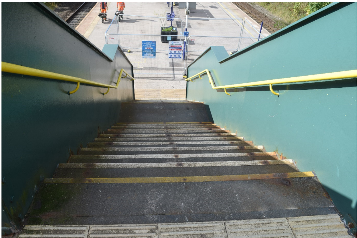
Photograph 6 – View from footbridge onto island platform
